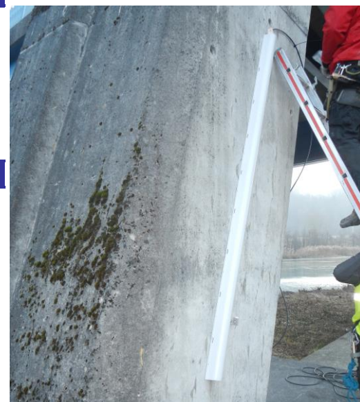
Optical Strand on a pylon leg
