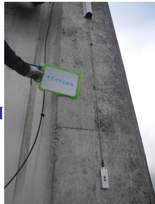
Optical Strand on the pylon upper part
